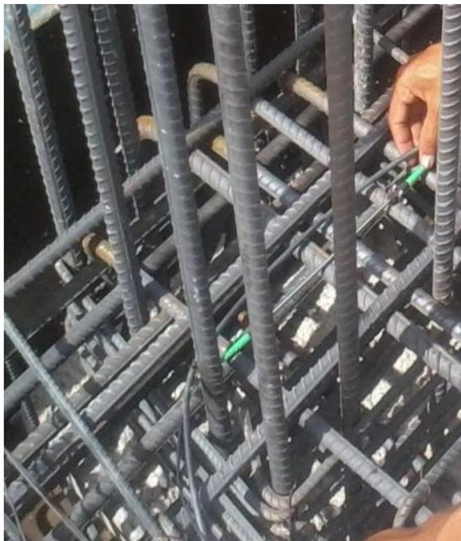
Figure 5. Installation of FBG sensor in a typical steel reinforced concrete structure
